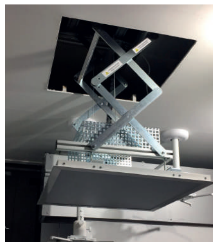
In the pictures below, examples of a false-ceiling installation of the V-LIFT bracket
